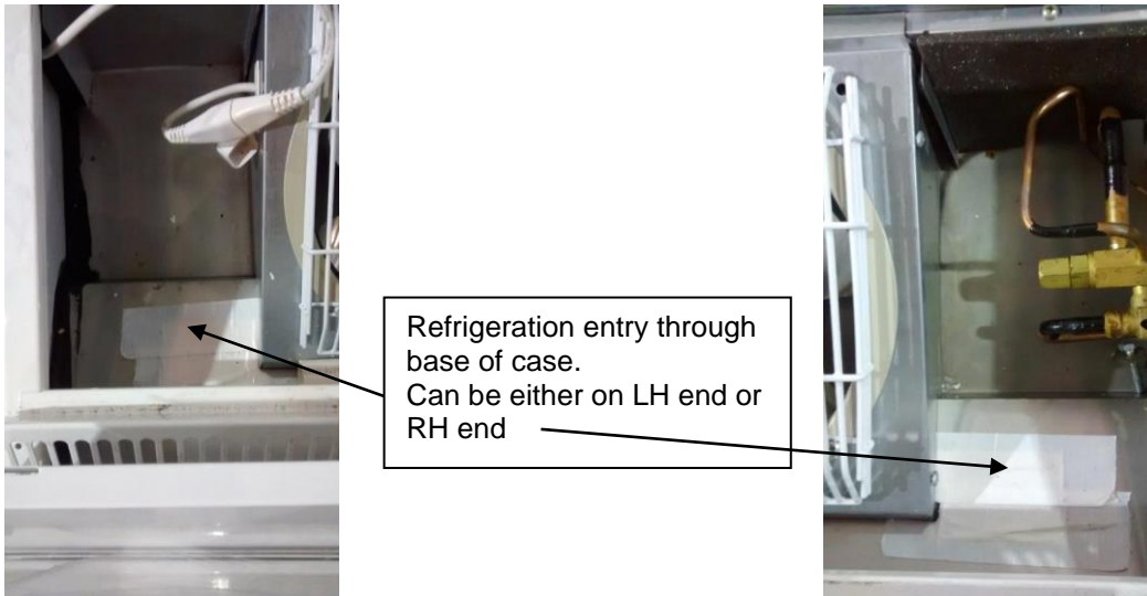
Figure 16:- Refrigeration connection
