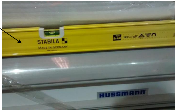
Figure 4:- Case levelling
